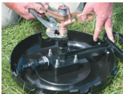
Screw the 20mm sprinkler into the socket.
