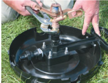
Screw the 20mm spinkler into the socket.
